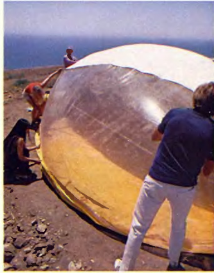
Weekend pied-à-terre or garden gazebo—the Pseudome's use expands to the limit of the imagination. Above, left to right: Once the base is filled, inflation begins. Then, as the bubble swells, the exterior is cleaned. Less than ten minutes later, the pad is ready for habitation.
