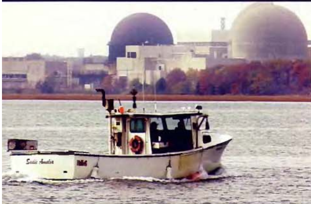
During the summer, boaters cruise past the domes. Zeh feels the riverfront is the plant's most vulnerable area.
