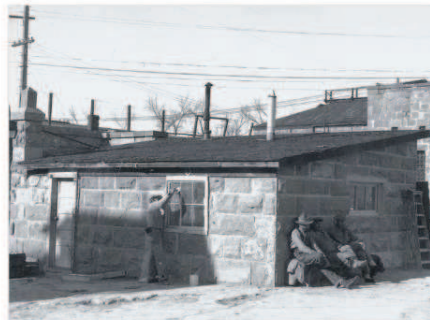
The nation’s first gas chamber, 1924.
